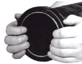
3. Gasket installation
