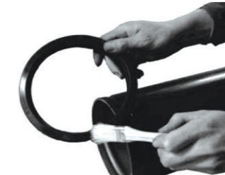
2. Lubricate gasket
