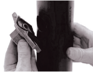
3. Gasket installation
