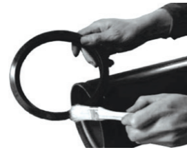
2. Lubricate gasket
