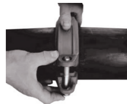
5. Housing installation
